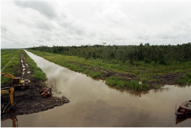
View of canals excavated in peat forest for Mega Rice Project, Central Kalimantan, 1997
