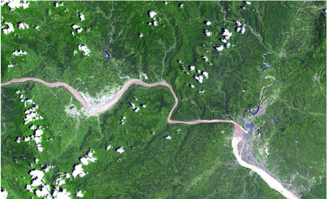
This ASTER image shows a 60 km stretch of the Yangzi river in China, including the Xiling Gorge, the most easterly of the three gorges. In the left part of the image is the construction site of the Three Gorges Dam, the world's largest dam.
