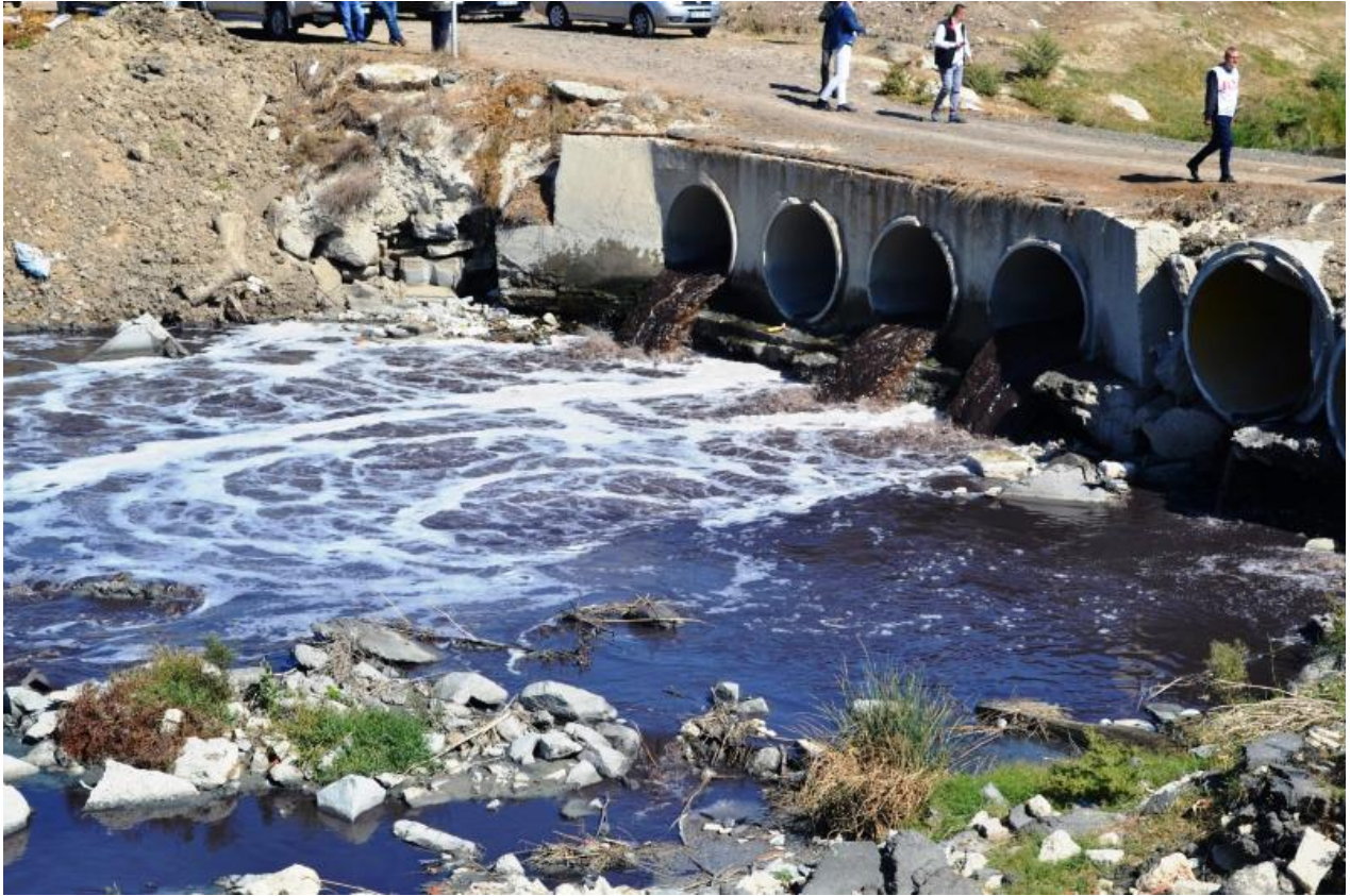
Industrial wastewater in the Ergene River.
