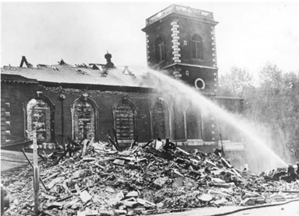
St. James's Piccadilly after the church had been bombed during the Blitz on 14 October 1940.
