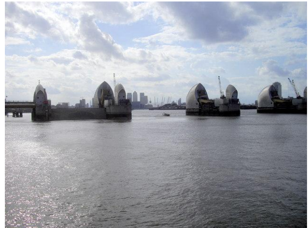
The Thames Flood Barrier
