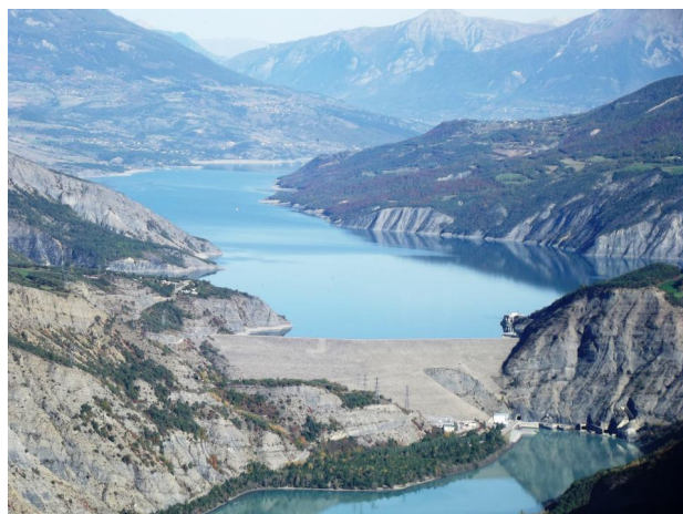
The Serre-Ponçon dam and the lake in 2013 (looking upstream from the left bank)
