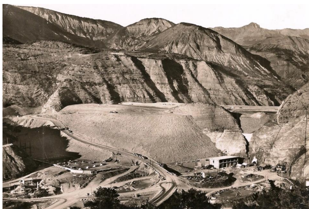
The embankment's construction (rock fill with an impermeable clay core) in 1958 (looking upstream from the left bank). One can see the future power plant house at its base.
